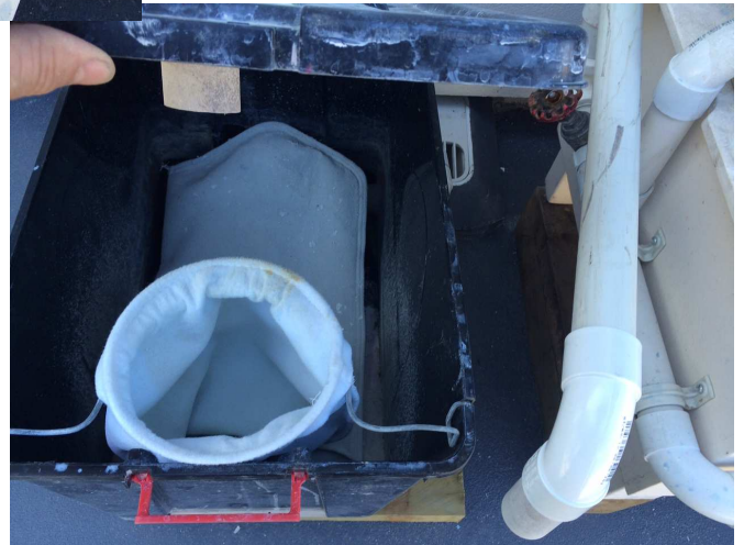
Pic 3 enviro - waste filter sock And discharge to drain
