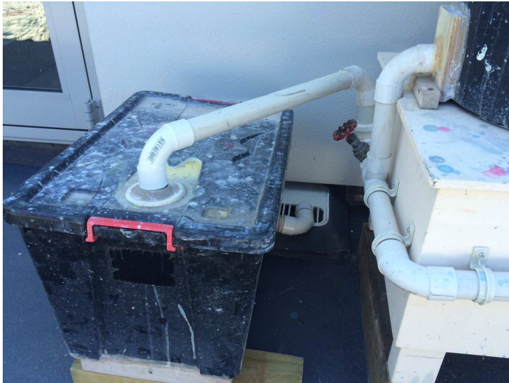
Pic 2 Raised height drains with stick plugs are in both holding tanks Separated paint sludge remains below drain level when emptied.
