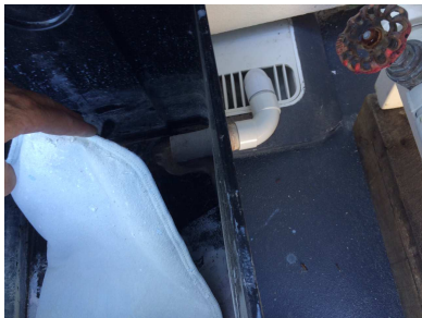
Pic 3 enviro - waste filter sock And discharge to drain
